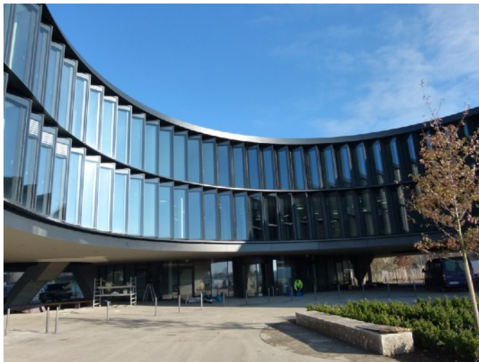
View of the new addition of the ESO Headquarters by Auer and Weber. Credit Claudia Neeser
